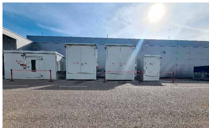
In special filling stations, solvents are dispensed in doses and unnecessary additional consumption is avoided.
